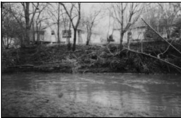
Redwood River eroding bank before the gabion project.
