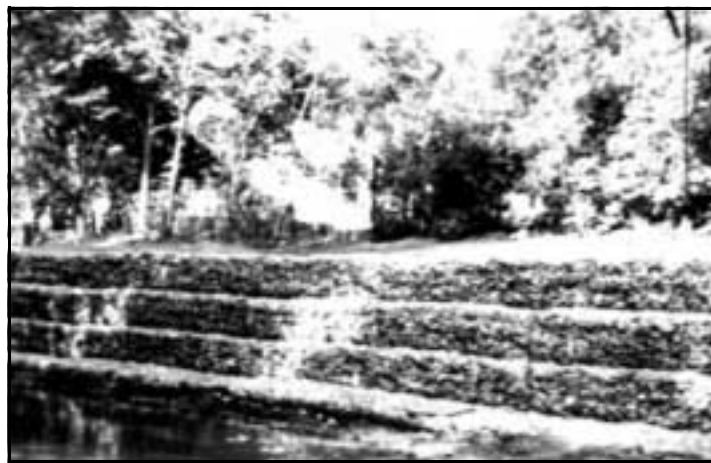
Completed gabion wall on the Redwood River.
